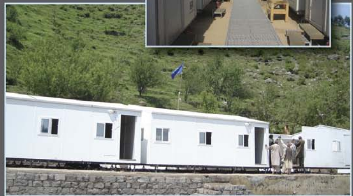
Photo: D&D - FRB (Fast Response Building)
