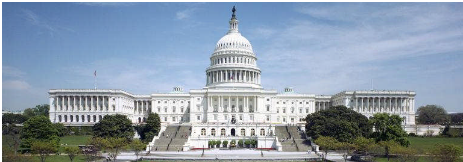
U.S. Congress, Credit: Architect of the Capital
